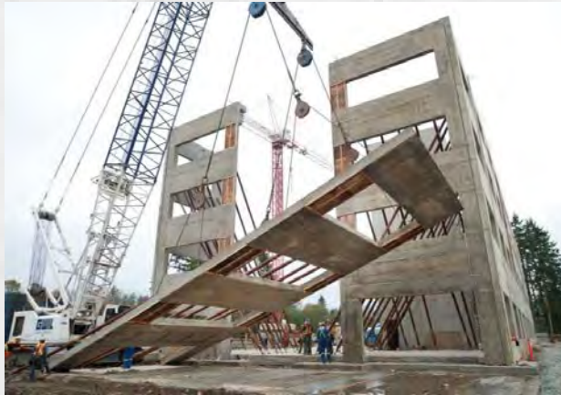
Tilt-up Concrete Walls
